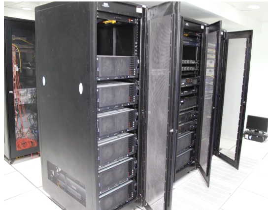
Figure 12: Blade Chassis
