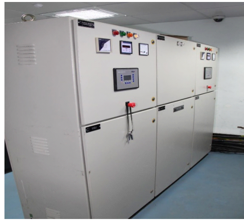
Figure 9: DG Synchronized Panel
