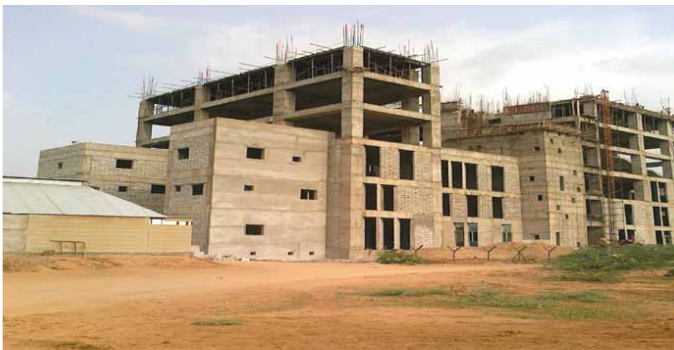
Fig. 1: INFLIBNET Centre's Building under Construction
